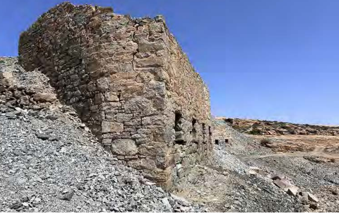
Cornish-built ore shoots at the Tweefontein mine in Concordia. Photo: Shannah Maree
